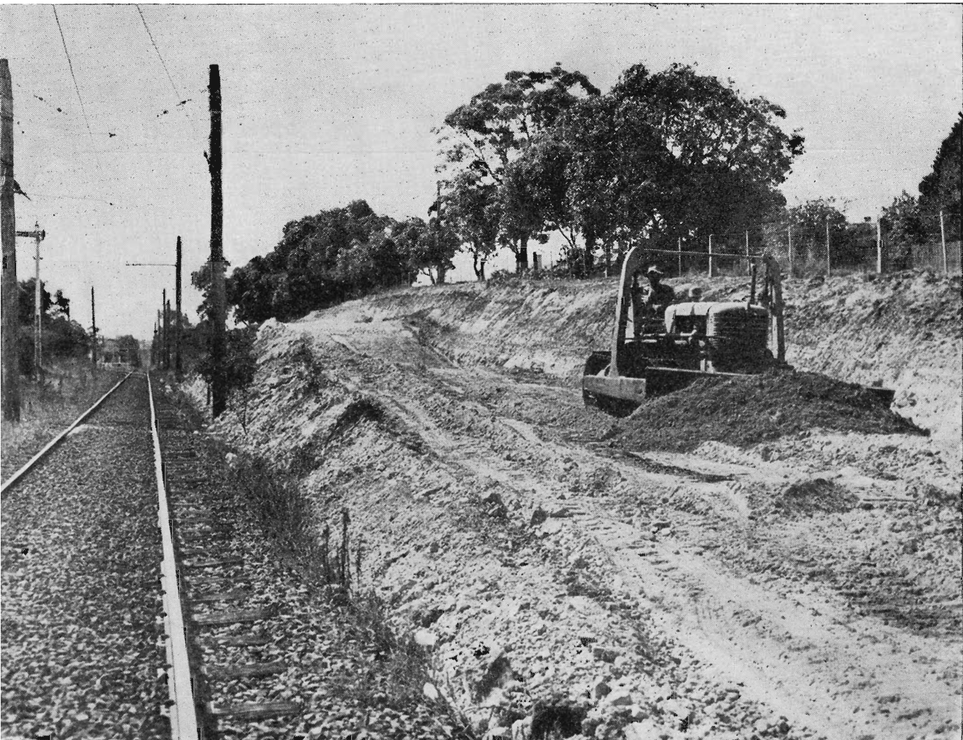
EXCAVATING FOR NEW TRACK, ASHBURTON LINE
